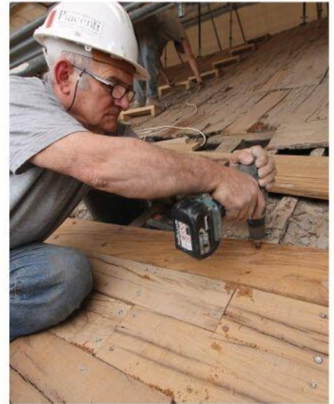
Restoration of the wooden boards
