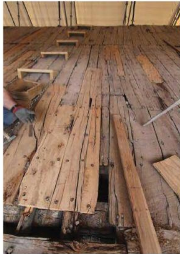
Restoration of the wooden boards
