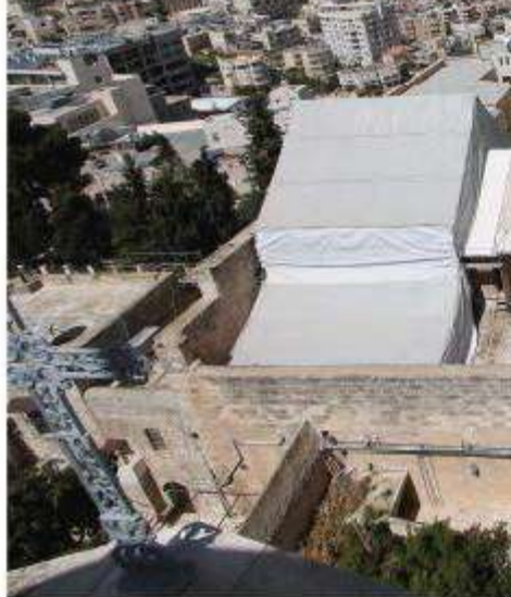
Roof conditions before restoration
