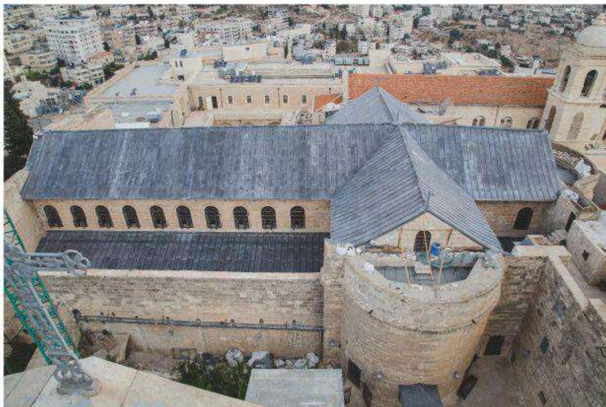
New roof after restoration
